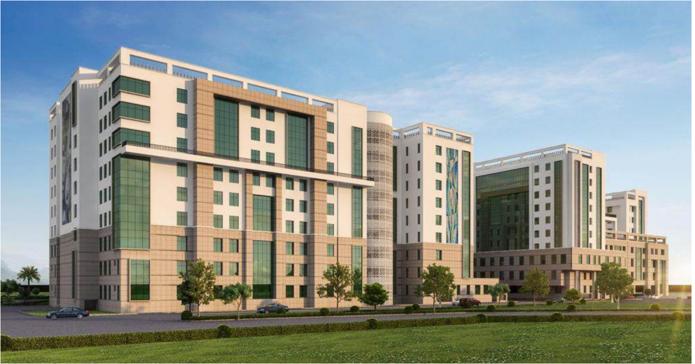
At the Mother and Child Block at AIIMS, New Delhi, we integrated biophilic design principles to foster a healing environment through natural connections and greenery.
