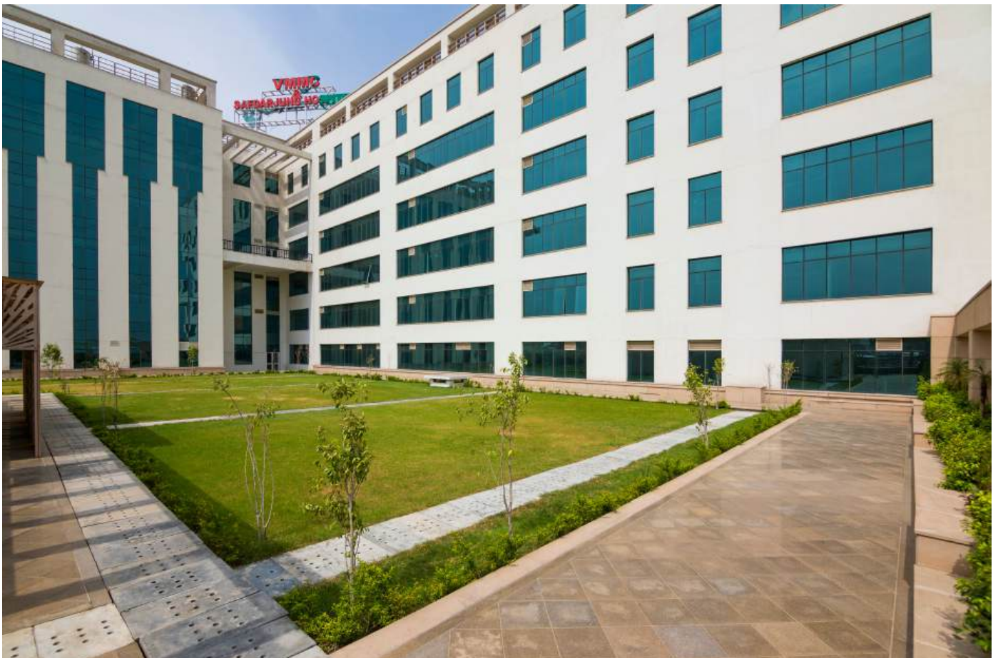
As part of Safdarjung Hospital's redevelopment in Delhi, the New Emergency Block was designed to enhance patient experience and streamline emergency care delivery.
